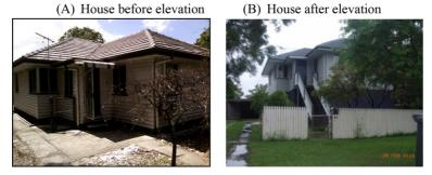
Figure 3: Example of elevating floor levels.
