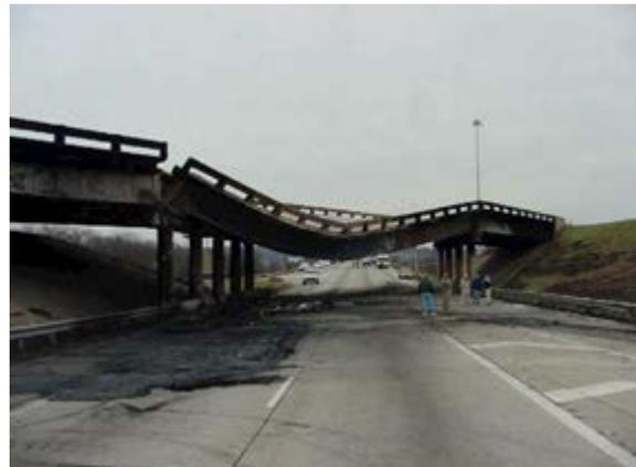
FIGURE 23: FIRE - CONCRETE BRIDGE [101]
