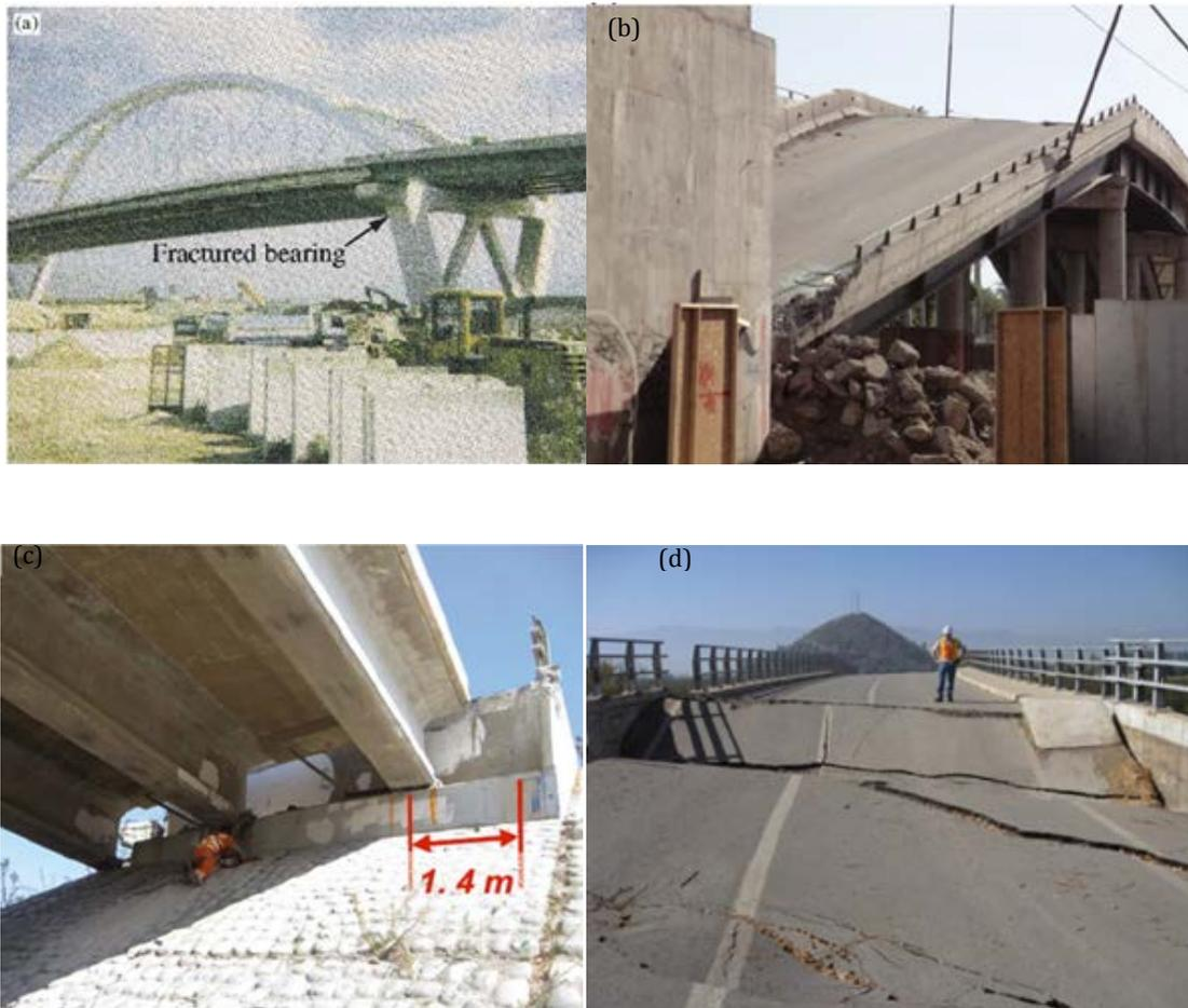
FIGURE 21: (A) FRACTURE OF BRIDGE BEARING OF NIELSEN BRIDGE TYPE DUE TO HANSHIN-AWAJI EARTHQUAKE
