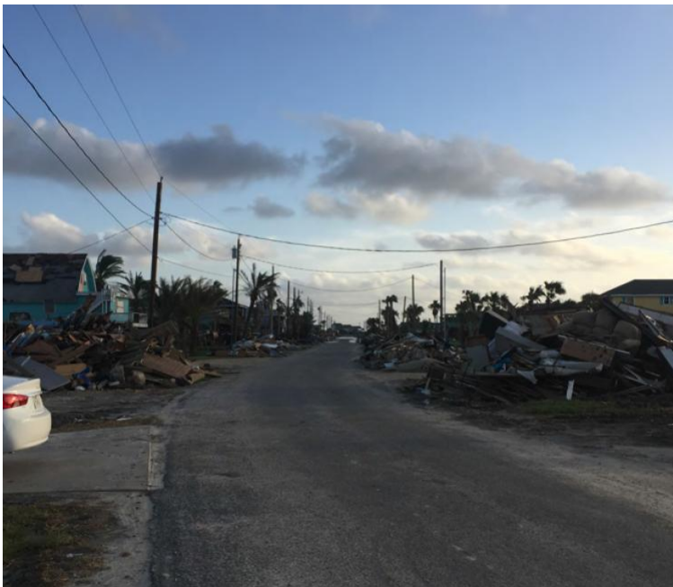
Harvey damage assessed by team CYCLONE, ENGINEERING
