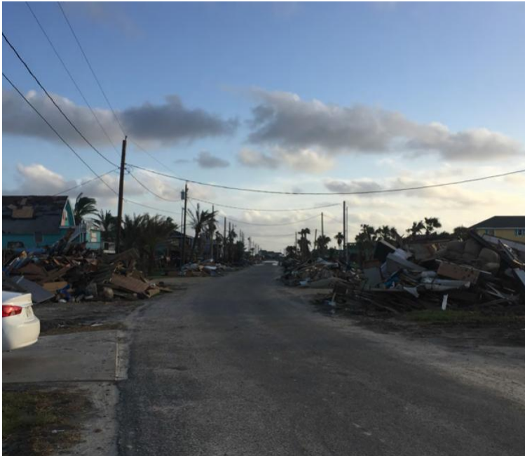
Harvey damage assessed by team CYCLONE, ENGINEERING
