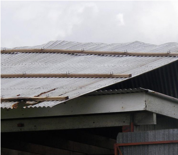
Failures on re-roofed houses CYCLONE, EXPOSURE
