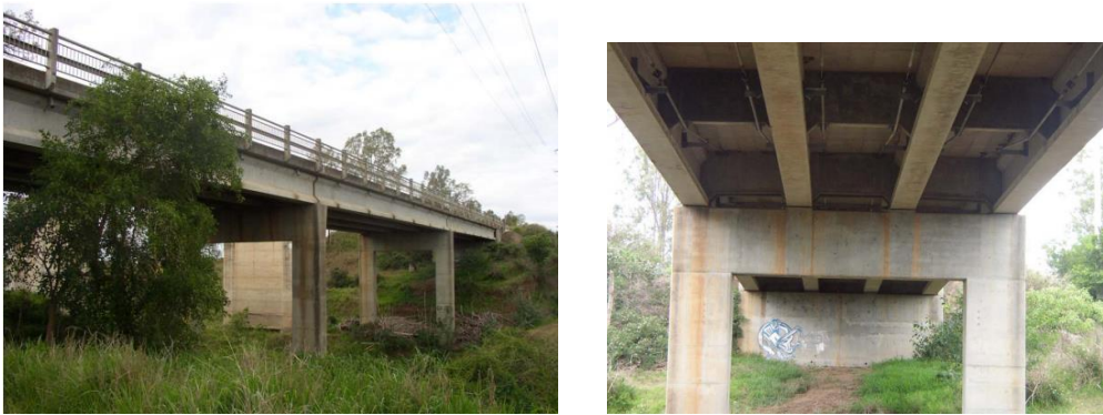
FIGURE 2.5: PHOTOS OF THE TENTHILL CREEK BRIDGE
