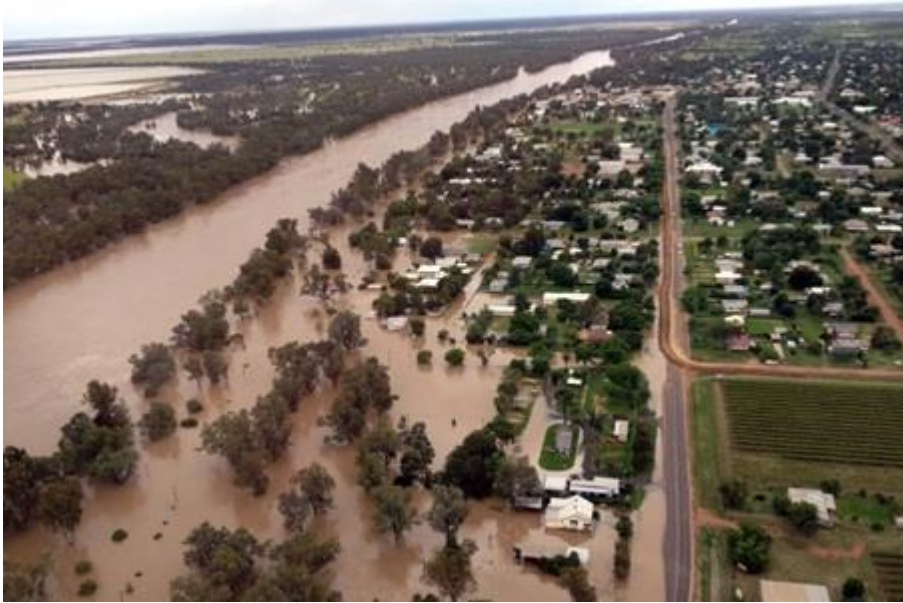
Figure 2: The 2012 flood in St George (ABC News, 2012a, 7 February) Three floods between 2010 and 2012 inundated similar sections of the town.
