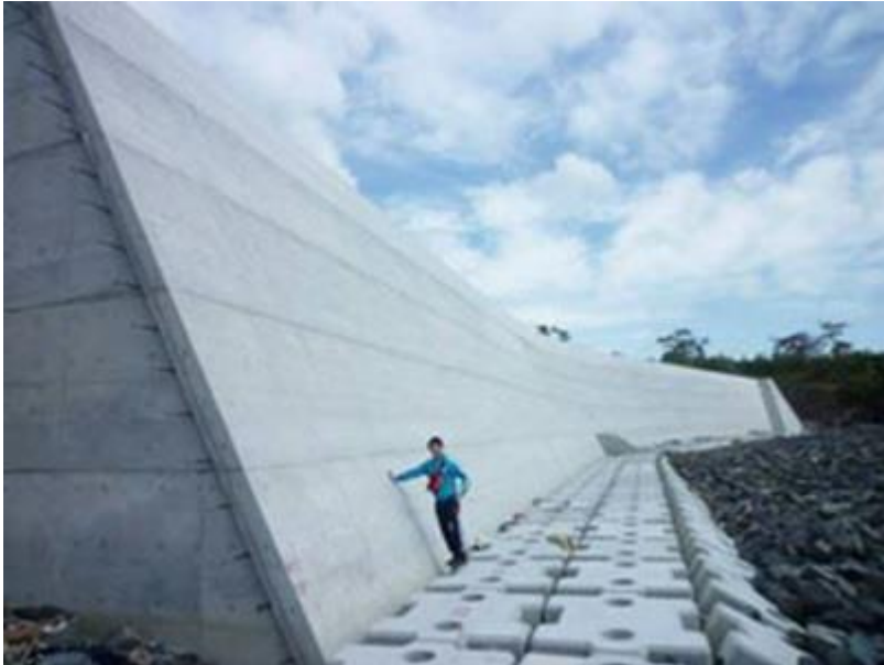
Figure 15: Tsunami levee near Koizumi at 9.8 m (Yomiuri Shimbun, 2014, 8 September)
