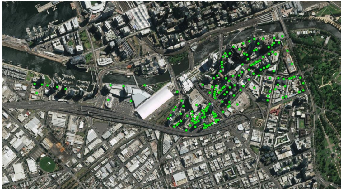
Figure 5: Buildings surveys in the Southbank business district survey with the capture of engineering parameters to enable mapping of earthquake vulnerability.
