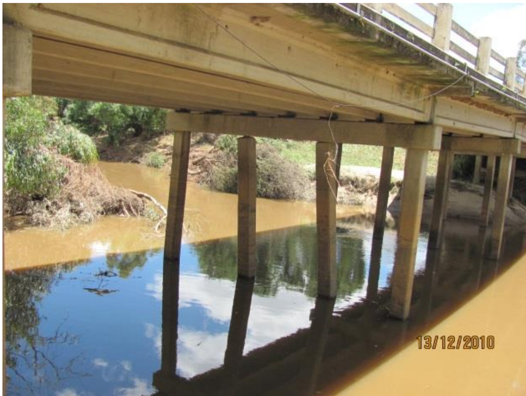
Figure 1-4: U-Slab Bridge Located in Victoria, Australia
