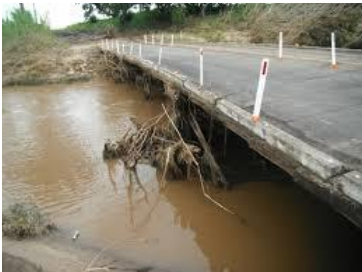
Figure 7-2 The damaged Thistlethwaite Bridge after the 2013 floods
