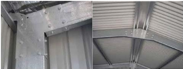
Typical cyclone rated shed knee bracket (left) and apex bracket (right)
