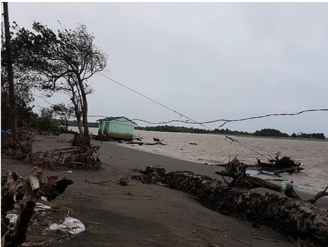
A damaged house in Aparri
