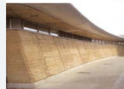
Small windows with protective overhang placed at the wall and roof junction, on the side facing a bushfire threat, reduces both potential ember entry and earthquake damage while encouraging greater internal air flow. Image from: Walker, P. (2005) Bermed earth - design and construction guidelines
