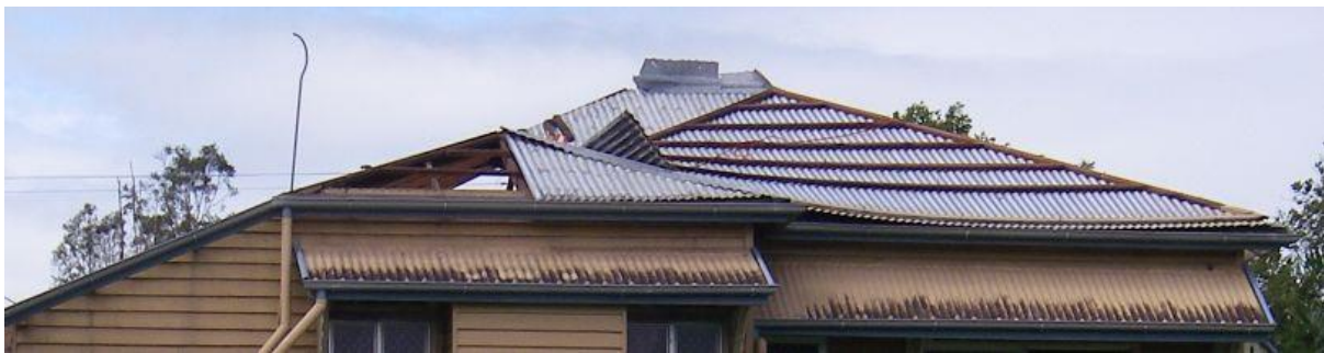
Figure 2. Part of the roof cladding with battens still attached flipped on to the leeward side
