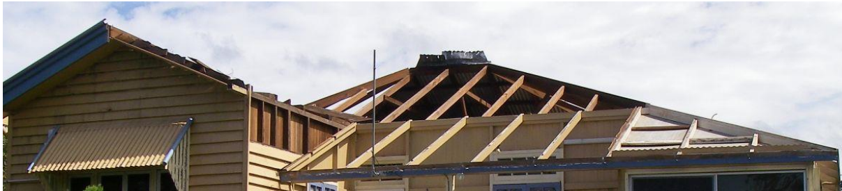
Figure 2. Part of the roof cladding with battens still attached flipped on to the leeward side
