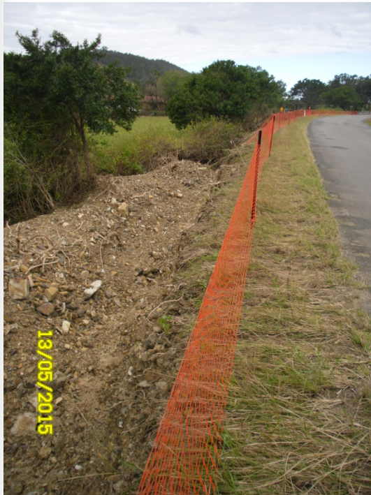
(A) Approach embankment
