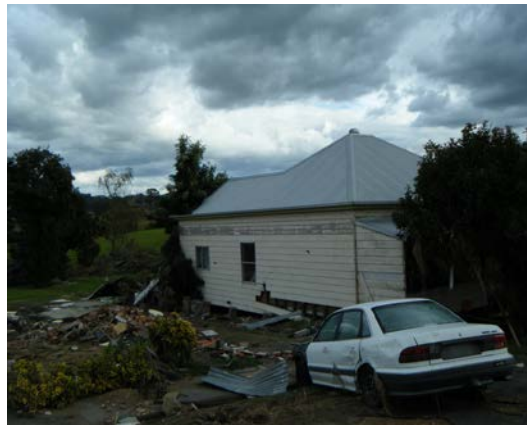
(4) severely damaged and moved off
