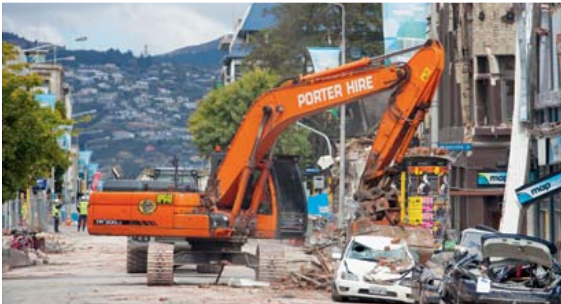
PHOTO: JOHN MCCOMBE, NEW ZEALAND FIRE SERVICE
