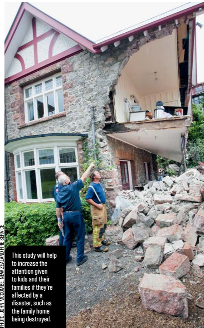
PHOTO: JOHN MCCOMBE, NEW ZEALAND FIRE SERVICE.
