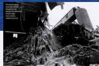
An elevator gantry crashed through the roof, pictured here above tonnes of raw, burnt sugar.
