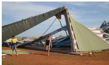
Damaged Building in Northern WA during Cyclone Christine, 2013.
