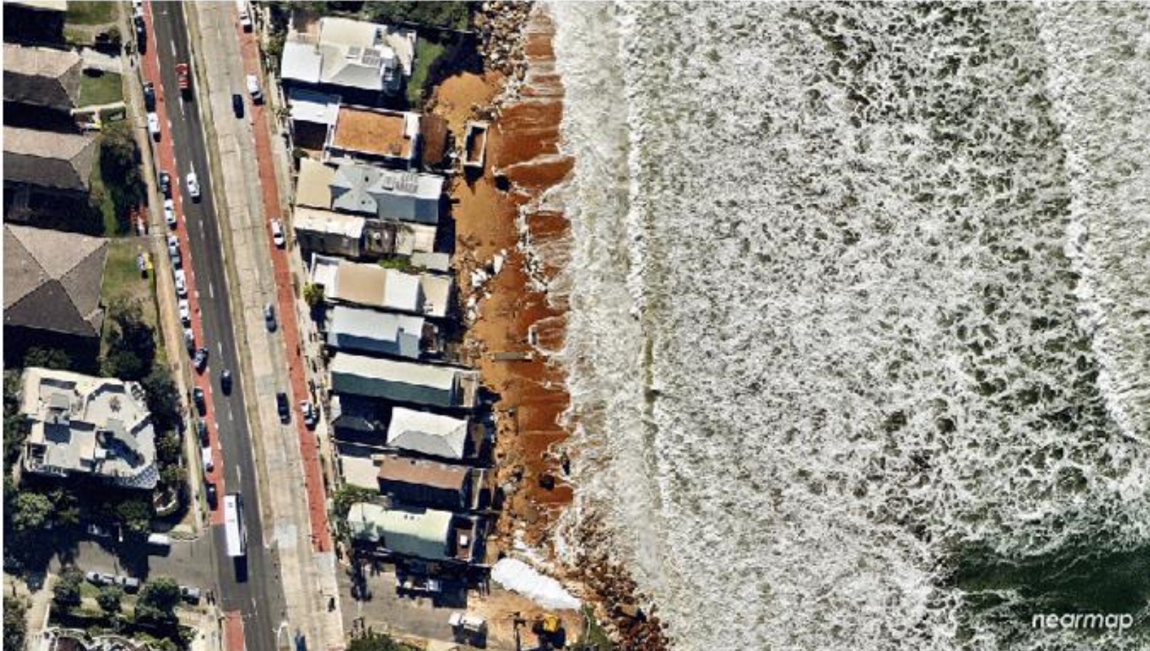
Before and after: a low pressure cell leaves Sydney's Collaroy beach devastated. (Nearmap)
