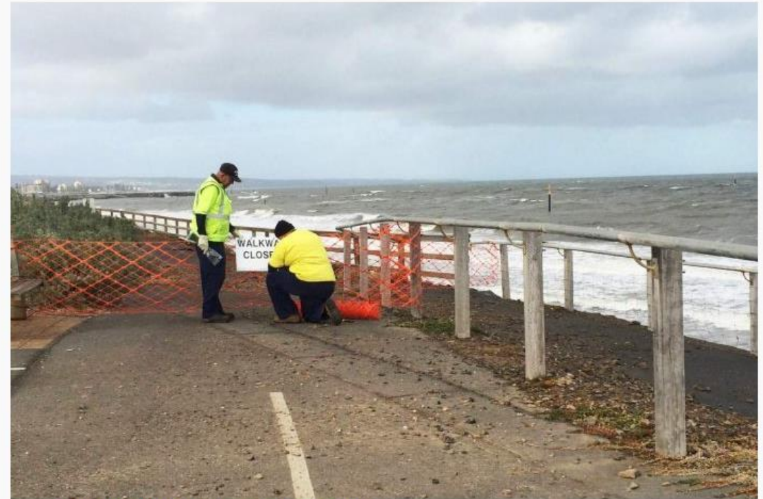
PHOTO: Storm damage has left little access to West Beach in Adelaide. (Supplied: City of Charles Sturt)
