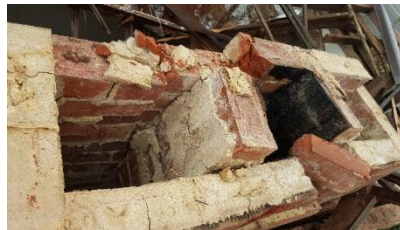
A chimney cross section
