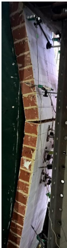
(a) Deflection profile at failure
