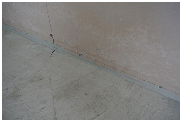
FIGURE 7: FILLING OF WALLS AND WALLS AND FLOOR CORNERS
