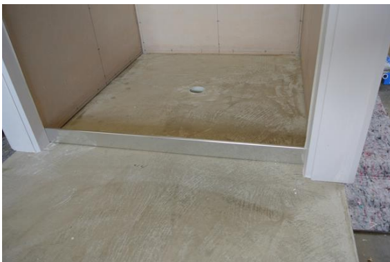
FIGURE 24: SHOWER SEAL FITTED TO ENTRANCE OR ENCLOSURE
