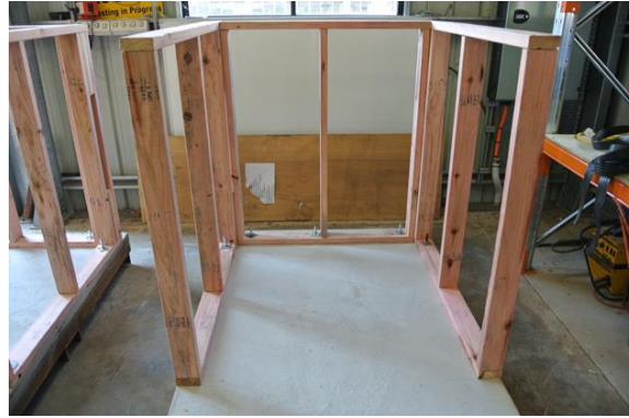
FIGURE 3: TWO LATERAL AND ONE END STUD WALLS
