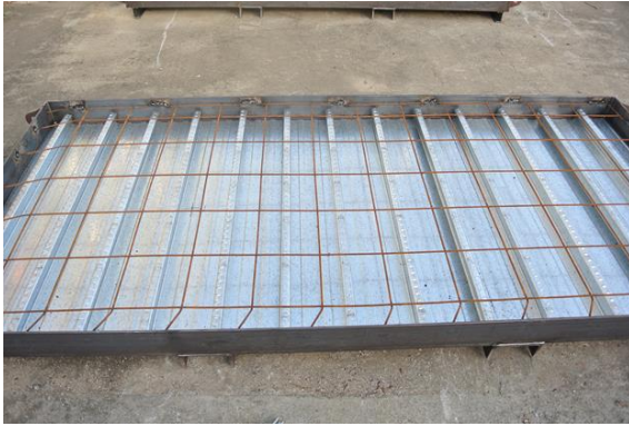
FIGURE 2: STEEL BED FOR CONCRETE SLAB
