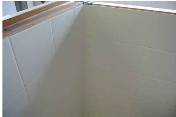
FIGURE 17: GAPS FILLED WITH SILICONE
