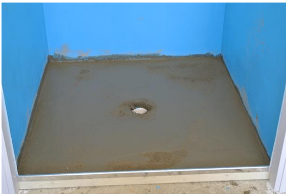
FIGURE 28: SHOWER ENCLOSURE RECESSED
