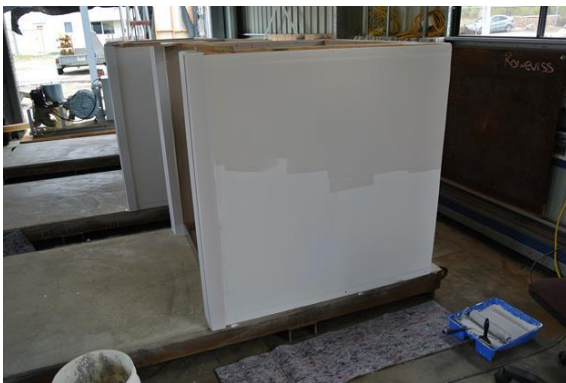
FIGURE 6: PAINTING OF PLASTER BOARD
