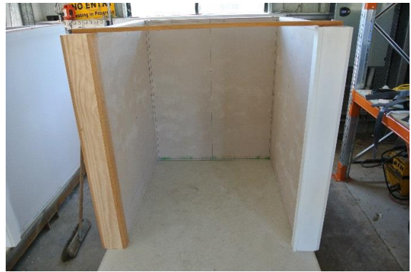
FIGURE 5: STUD WALLS LINED AND DOOR JAMBS INSTALLED
