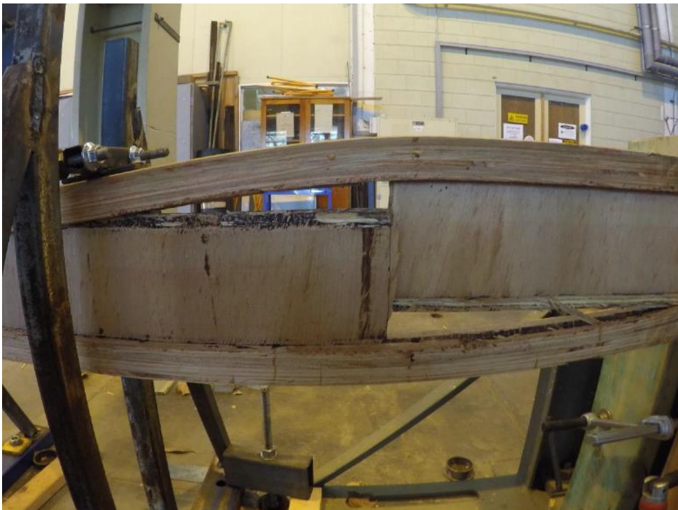
FIGURE C20: FAILURE OF H2 TREATED TIMBER T SECTIONS WET-DRY SAMPLES: BOTTOM FLANGE RUPTURE AND WEB DISLODGED FROM FLANGES
