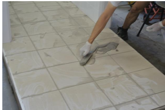
FIGURE 15: TILES GROUTING
