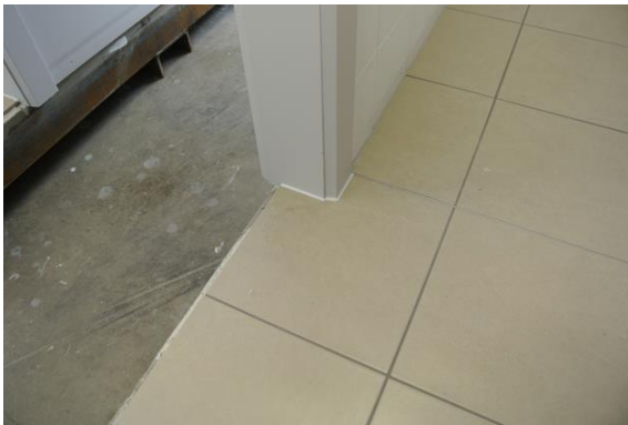
FIGURE 16: GAPS FILLED WITH SILICONE
