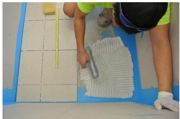
FIGURE 9: FLOOR TILING
