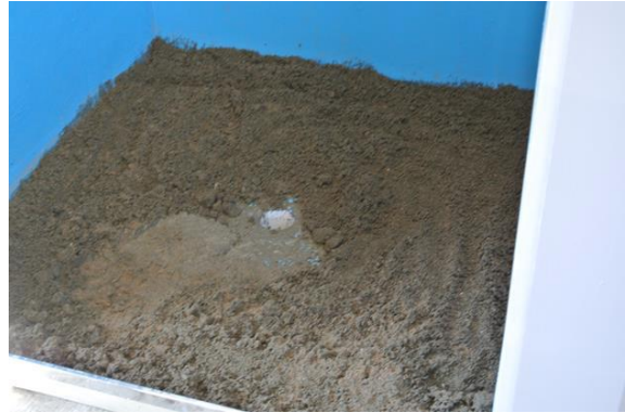
FIGURE 27: RECESSING OF SHOWER ENCLOSURE
