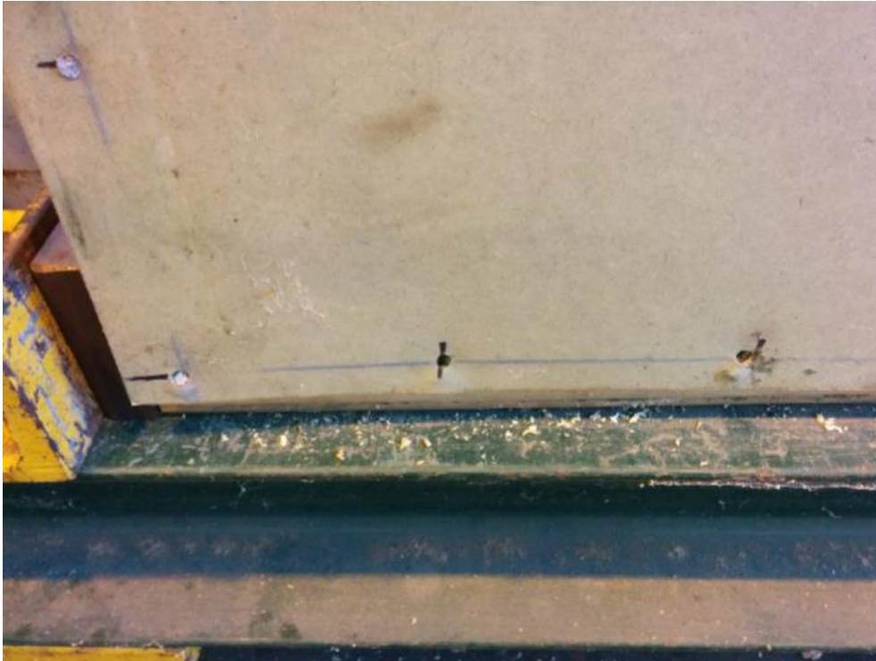
FIGURE B19: NAIL FAILURE ON HDF (WET-DRY SAMPLES)
