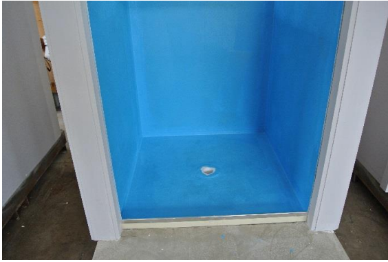
FIGURE 26: WATERPROOFING OF SHOWER ENCLOSURE
