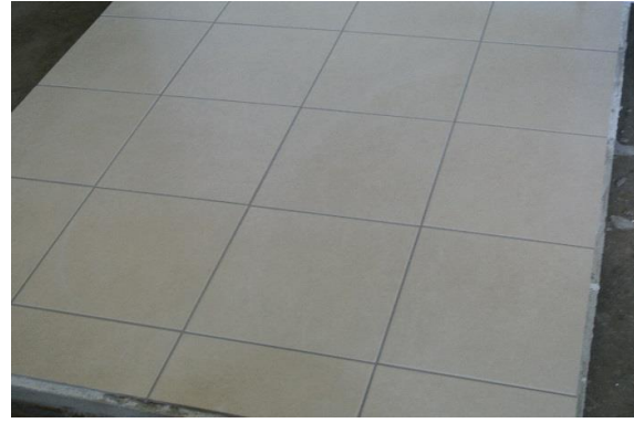
FIGURE 35: TILES GROUTING
