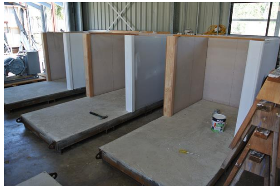
FIGURE 21: STUD WALLS LINED AND DOOR JAMBS INSTALLED
