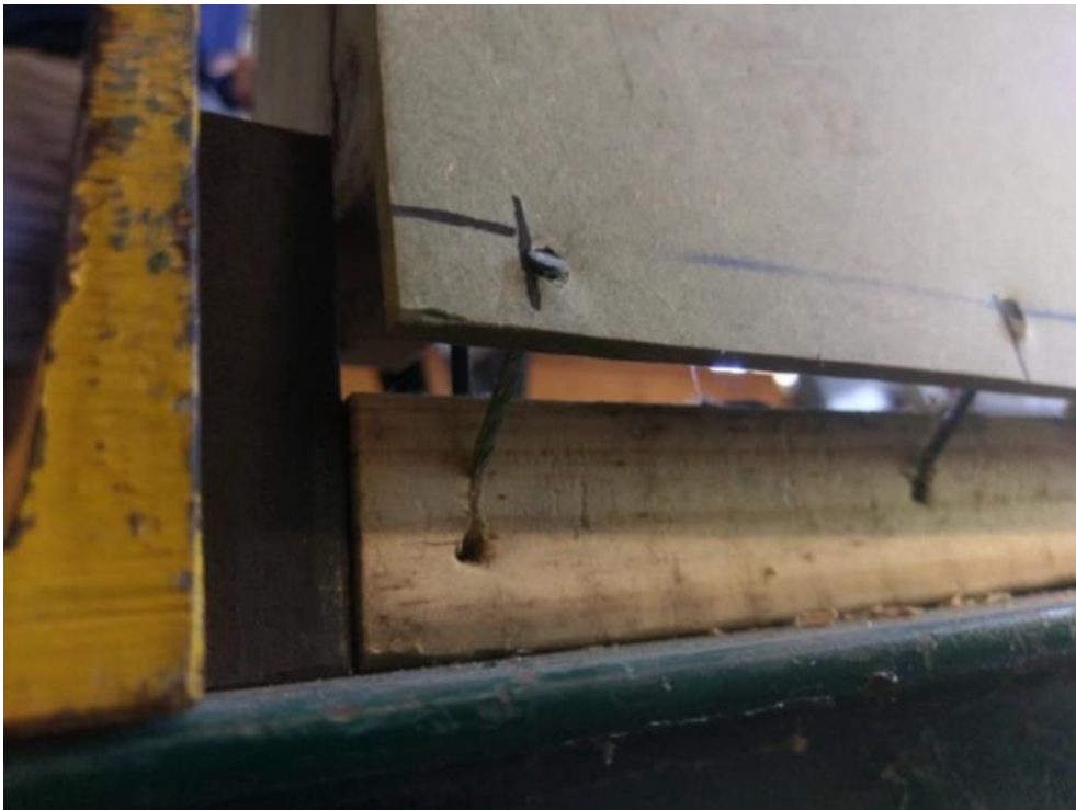
FIGURE B18: NAIL FAILURE ON HDF (WET-DRY SAMPLES)
