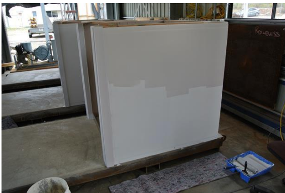
FIGURE 22: PAINTING OF PLASTER BOARD
