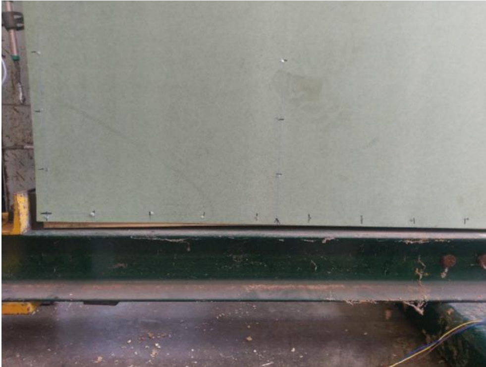
FIGURE B15: OSB BRACE SHEETING FAILURE (WET-DRY SAMPLES)
