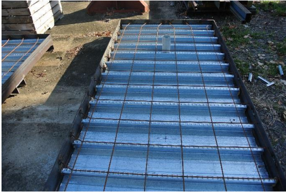
FIGURE 18: STEEL BED FOR CONCRETE SLAB WITH PVC PIPE
