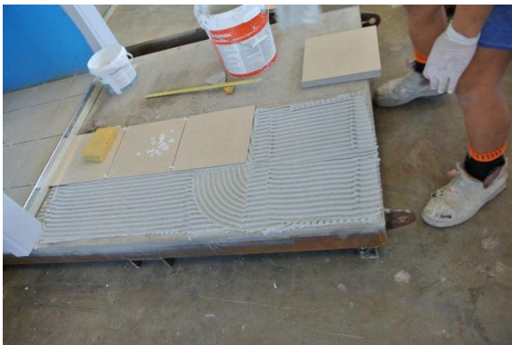
FIGURE 30: FLOOR TILING
