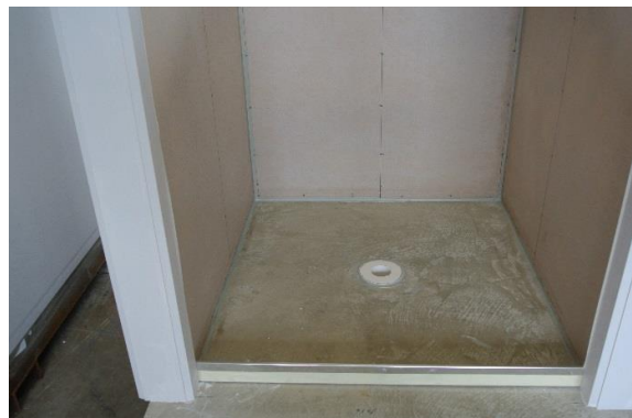
FIGURE 25: FILLING OF CORNERS BETWEEN WALLS AND FLOOR
