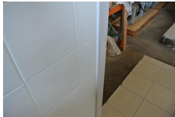
FIGURE 37: GAPS FILLED WITH SILICONE
