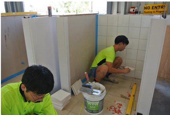
FIGURE 12: WALL TILING
