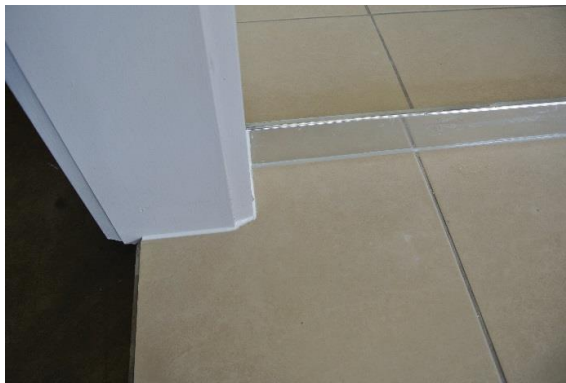
FIGURE 36: GAPS FILLED WITH SILICONE
