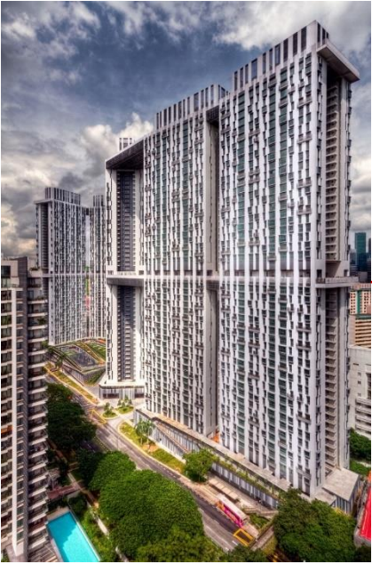
High Rise Residential Buildings
