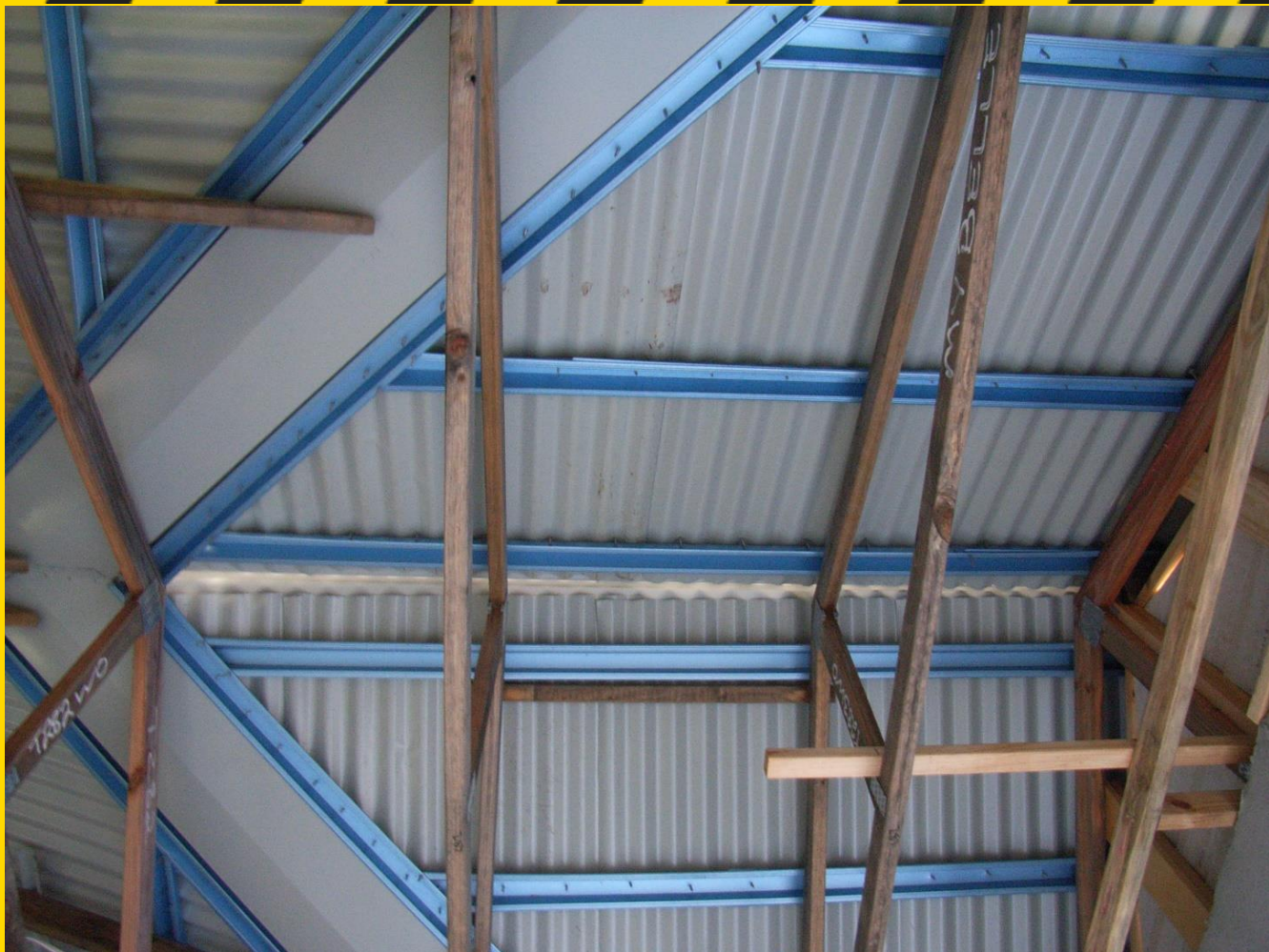
Roof Structure of a House under construction
