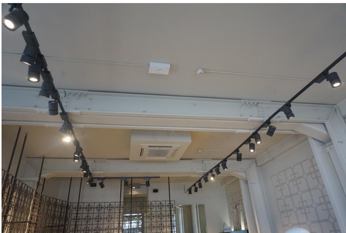
Figure 1: Ground floor view of retrofitted two storey retail structure of the 1930s period in Napier, New Zealand. The building is of poorly detailed reinforced concrete frame construction with unreinforced masonry infill walls. Ductile steel moment frames have been retrofitted to strengthen the structure in the transverse direction.
