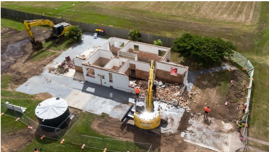
VHBB home demolition, April 2023 – Photo courtesy of QRA
