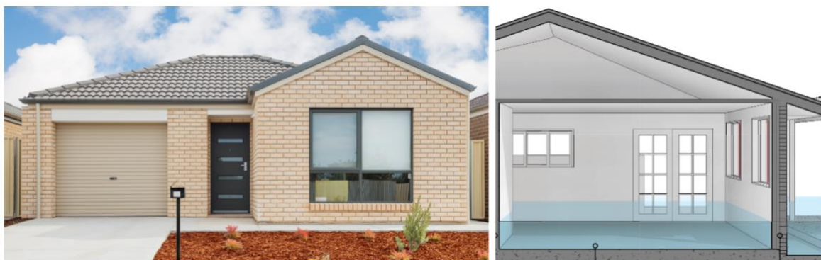
Example of a slab-on-ground with brick veneer wall system – Photo courtesy of Adobe Stock and QRA
