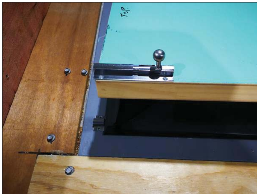
Figure 12: Trial SS4 Top Barrel Bolt Undamaged
