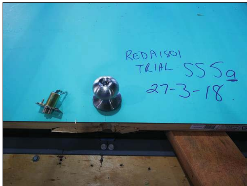
Figure 20: Trial SS5a Broken Lock Mechanism and Damaged Door
